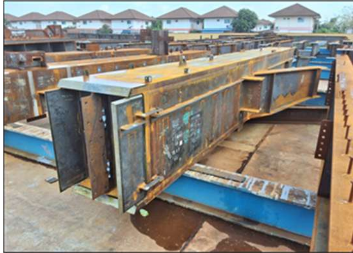
Example image of Beam work
